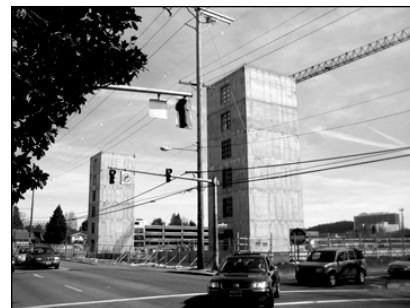
Providence building construction on Halsey in April
